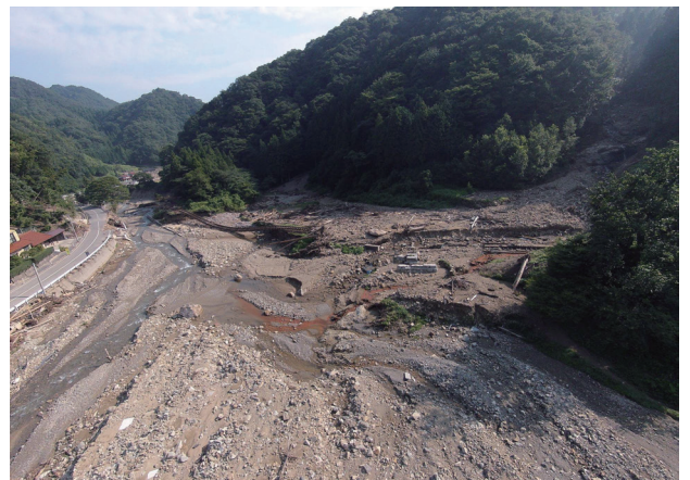
図 57 山口・島根豪雨災害空撮調査. 名賀川の河床氾濫(図 55 の点 B) Fig. 57 Aerial photo of a Naoyosih-river flood area caused by 2013 Yamaguchi-Shimane heavy rainfalls (at point B in Fig. 55).
