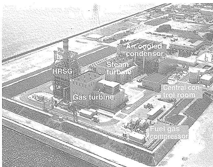
Fig. 2 Gas turbine combined cycle verification plant ("T" point) at Takasago Machinery Works
