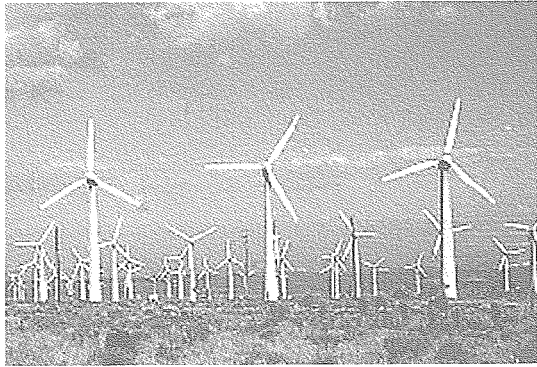
Fig. 4 Tehachapi wind farm in Cal., USA
