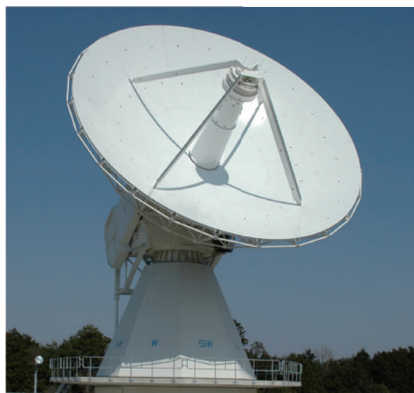
Fig. 3 Photo of the new antenna
