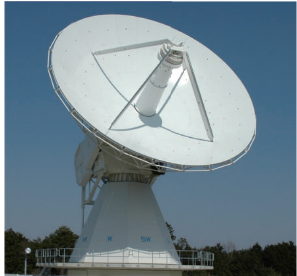
Fig. 3 Photo of the new antenna
