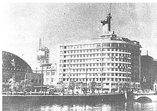
Photo 5 Complete view of Asahi Building in Osaka
